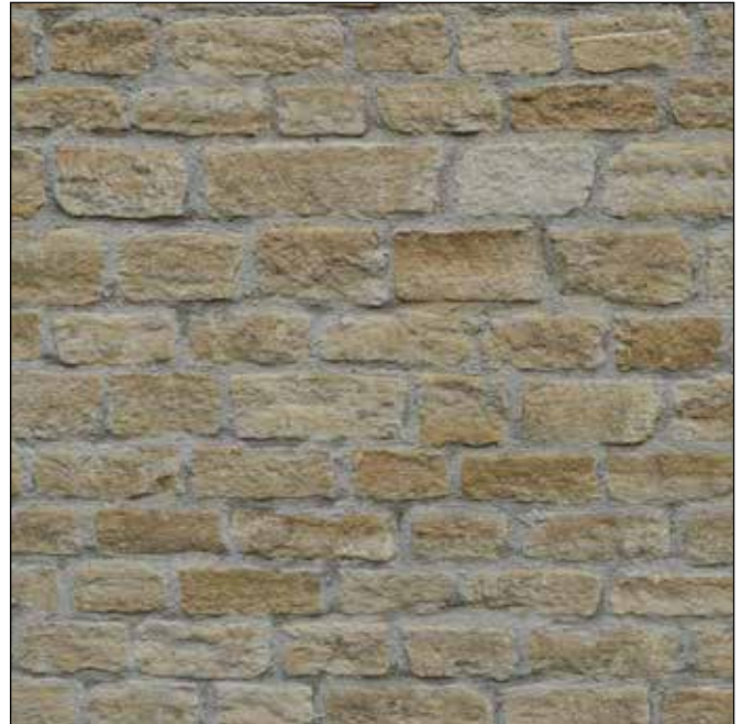
Fig. 3 Recent traditional mortared wall
