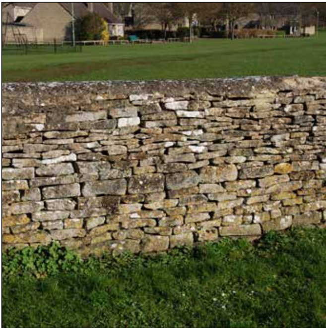
Fig. 1 Traditional dry stone wall
