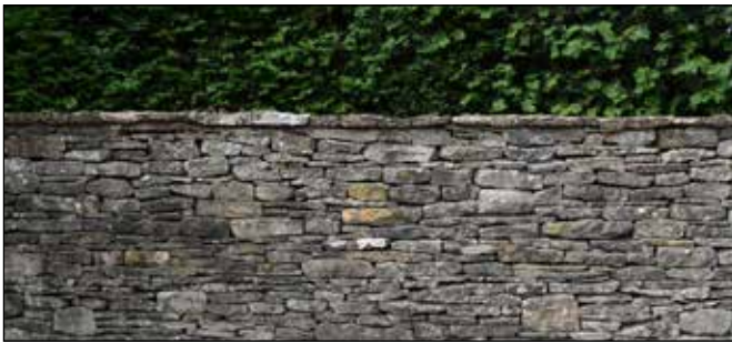
Fig. 3 Recent traditional mortared wall
