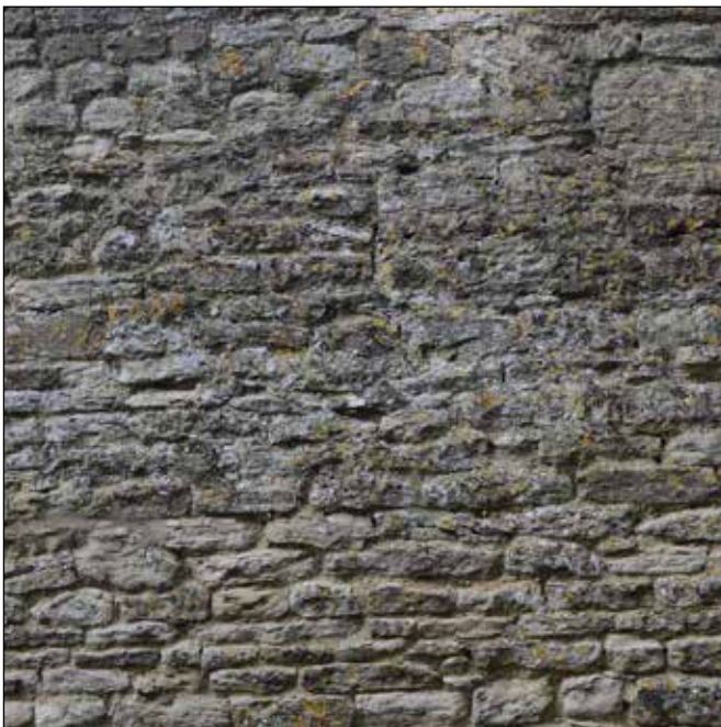
Fig. 4 Traditional rubble stone wall
