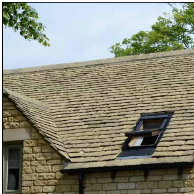
Fig. 7 Artificial stone slate roof with flush roof-light
