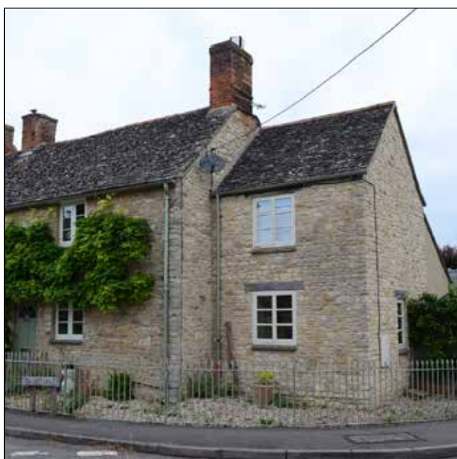
Fig. 1 Two-storey side extension to a traditional house
