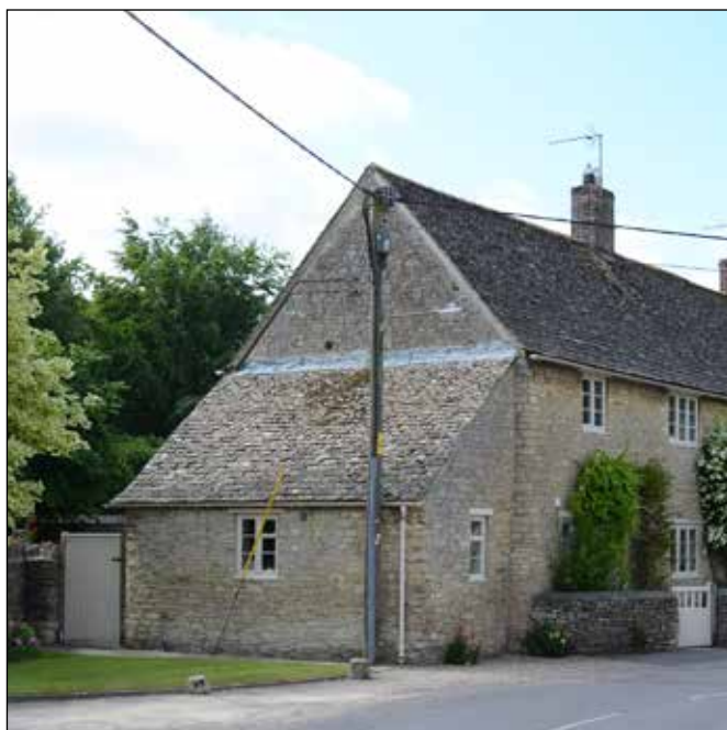
Fig. 4 Single-storey lean-to extension
