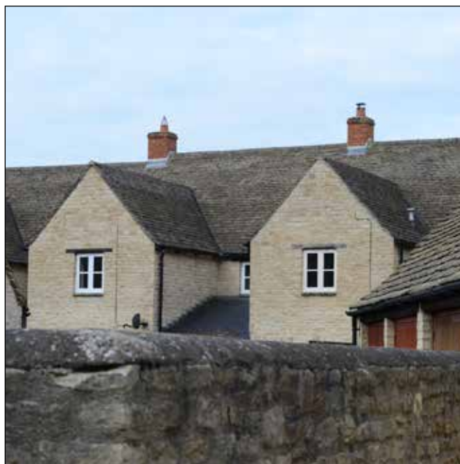
Fig. 3 Two-storey rear projecting gabled extensions
