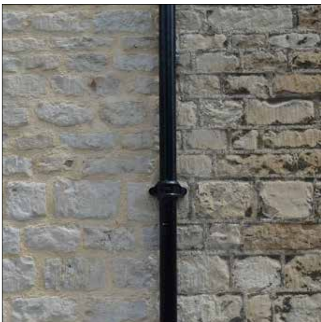
Fig. 8 Stonework should always be repaired with care
