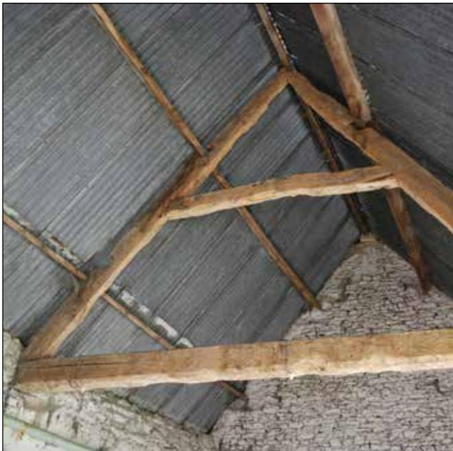
Fig. 7 Original roof trusses should be retained
